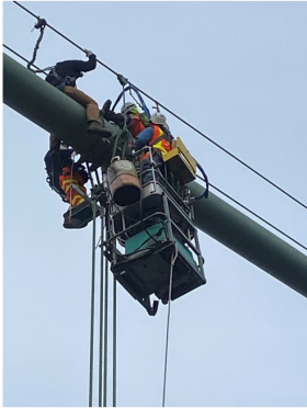
The old way with the spider. 3-4-person team on the cable, 1 operating the spider and 1 ground person.
