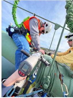
The new way. 3-person crew on the cable. All the equipment needed is carried by the crew attached with lanyards to their person. Almost everything needed is pictured in this photo.
